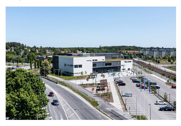
To achieve the desired effect, the black-and-white façade was designed using various materials, creating an exciting, organic pattern through perforations in the façade panels with holes of different sizes to soften the black concrete and large glass sections. The white, backlit, and perforated metal façade also provides a beautiful light variation throughout the day. The materials, colors, and details are thoughtfully designed for durability over time and to create pleasant environments.
