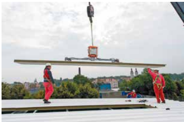
Pic. 8 and 9. Assembly of roof panels.
