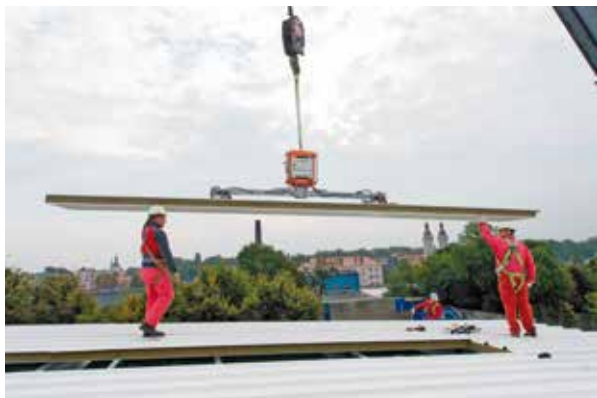
Pic. 8 and 9. Assembly of roof panels.
