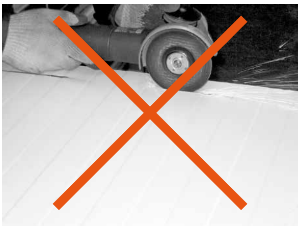
Pic. 6 and 7. Do not cut panels with angular grinding machine as anticorrosive covers can be devastated.
